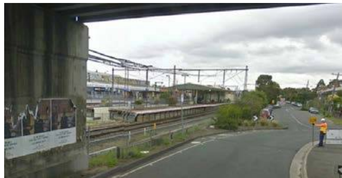
Figure 3: Burnley Station from beneath Burnley Street overpass
