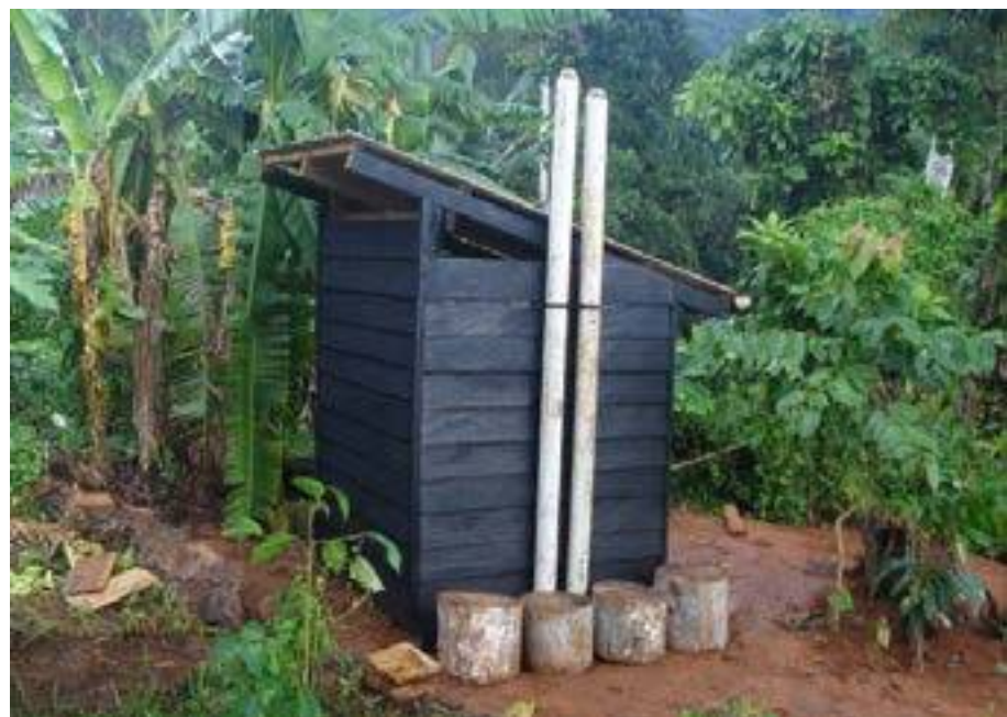
Figure 5: Completed latrine project
