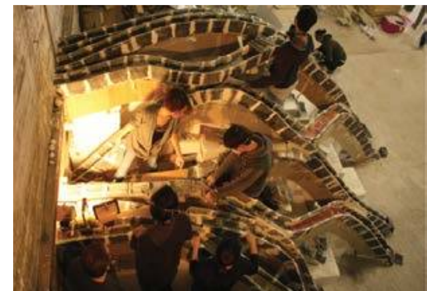
Figure 10. Aerial view of construction process for the ribs, demonstrating the laying of the tiles over the guidework. Photo: Jordan Soriot
