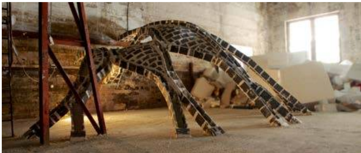
Figure 11: The completed 'Ribbed Catalan' tiled vault. Photo by Michael Ford_studio
