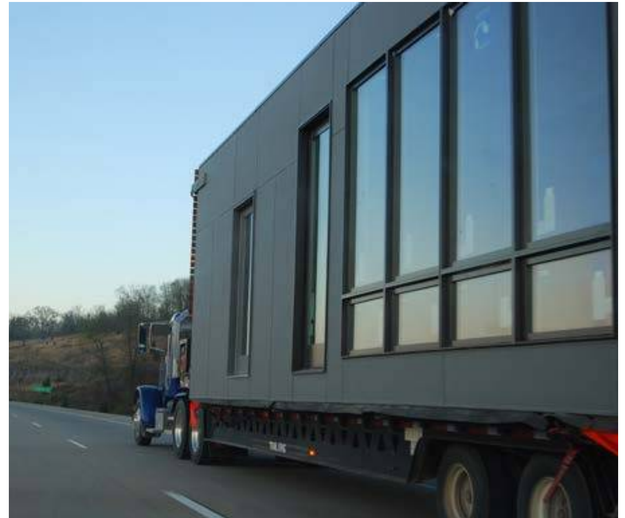
Figure 9: Prefab module in transit
