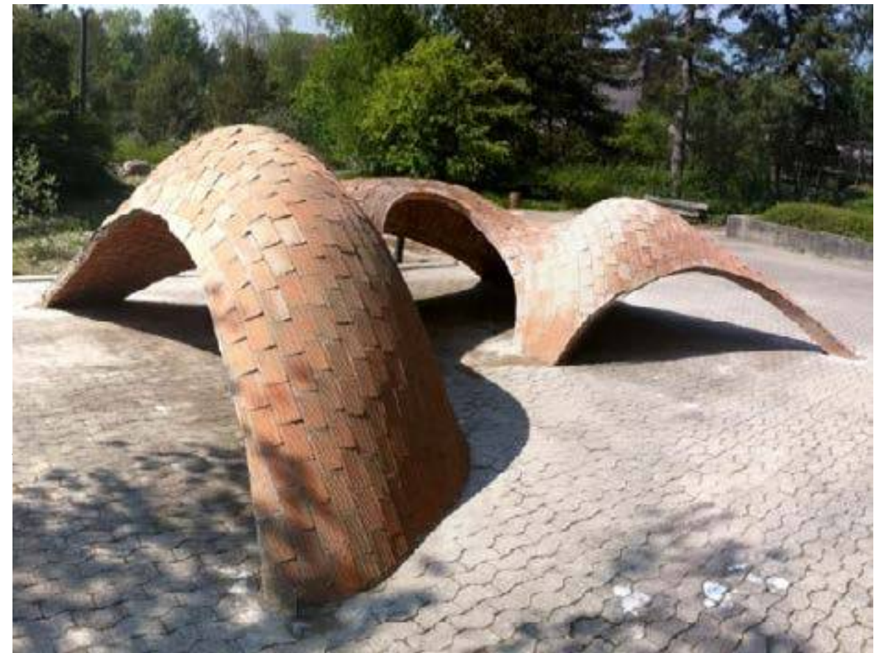
Figure 2: Freeform tiled vault built by Lara Davis (PhD research project) undertaken with the Block Research Group, ETHZ, 2011. Photo: Lara Davis.
