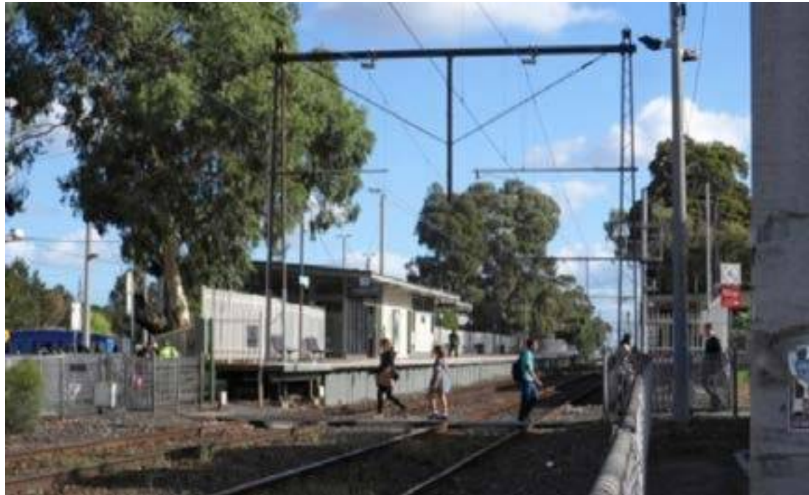
Figure 2: Reservoir station – the only pedestrian crossing place for several hundred metres
