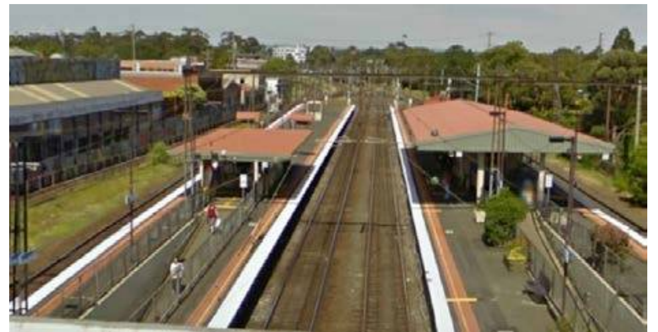
Figure 4: Burnley Station from Burnley Street overpass
